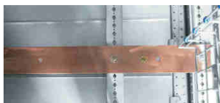
Main terminal consisting of a copper or aluminium bar.
