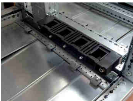
Fix the supports between the functional upright and the structural upright
