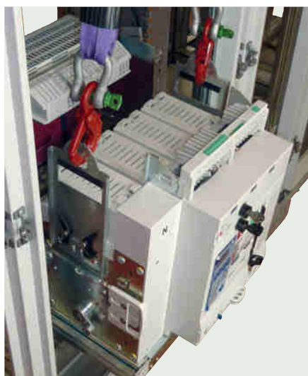
Installing a draw-out DMX 3 in its base.
