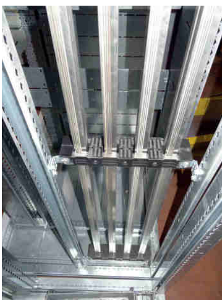
Position the busbars and tighten the supports to ensure the bars are held in place. (Tightening torque: see page 29).
