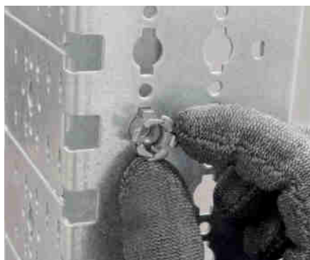
Fitting the clip-nuts
