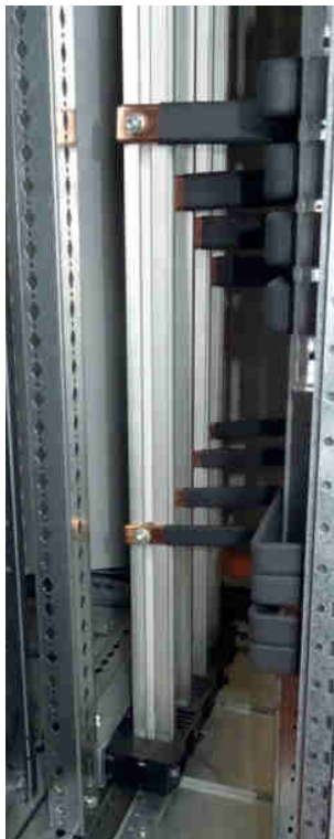
Busbar installed in cable sleeve.
